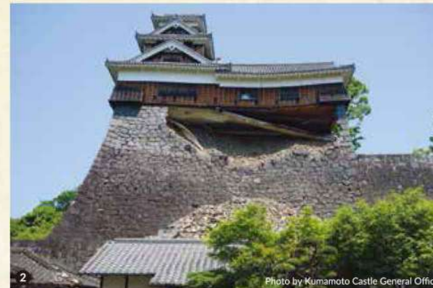
The lidamaru Five-Story Turret sustained considerable damage in the Kumamoto earthquakes. A single corner of the stone wall miraculously held out through the quakes to prevent a complete collapse of the turret.
