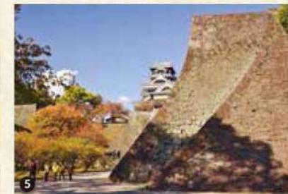
The lidamaru Five-Story Turret sustained considerable damage in the Kumamoto earthquakes. A single corner of the stone wall miraculously held out through the quakes to prevent a complete collapse of the turret.
